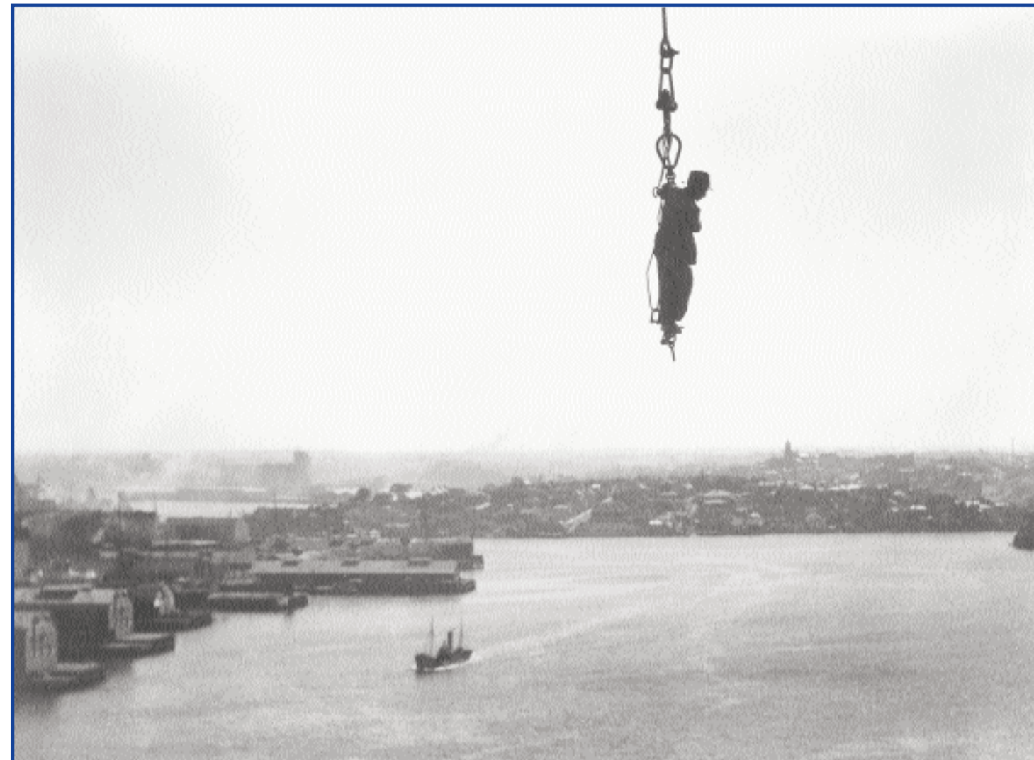
The practice of 'riding the hook' was eventually banned in NSW — the last State to do so — in 1983 after decades of campaigning. Photo: Henri Mallard, Riding the Crane , c1930? silver gelatin photograph. Courtesy of The Henri Mallard Collection, The Australian Centre for Photography.
