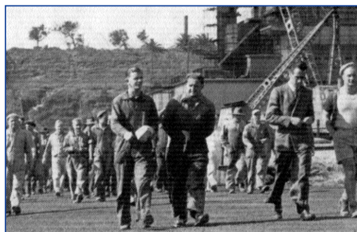
Bunnerong construction and power workers, with BWIU organiser Tom McDonald, walk out the gate in pursuit of site allowances in the early 1950s.
