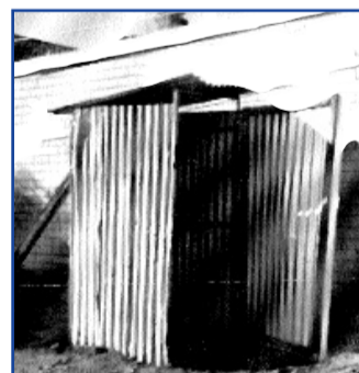
Bosses were still trying to get away with dunnies like this on building sites in the 1980s.
